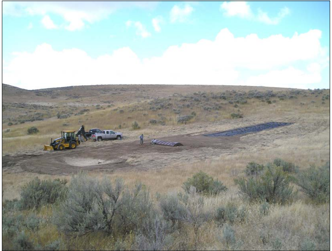
Southwest Region Fish and Game employees install a new 1,800-gallon guzzler on Charles Woodworth's CRP land for mule deer. Another one was also installed higher on the hill for upland game birds.
